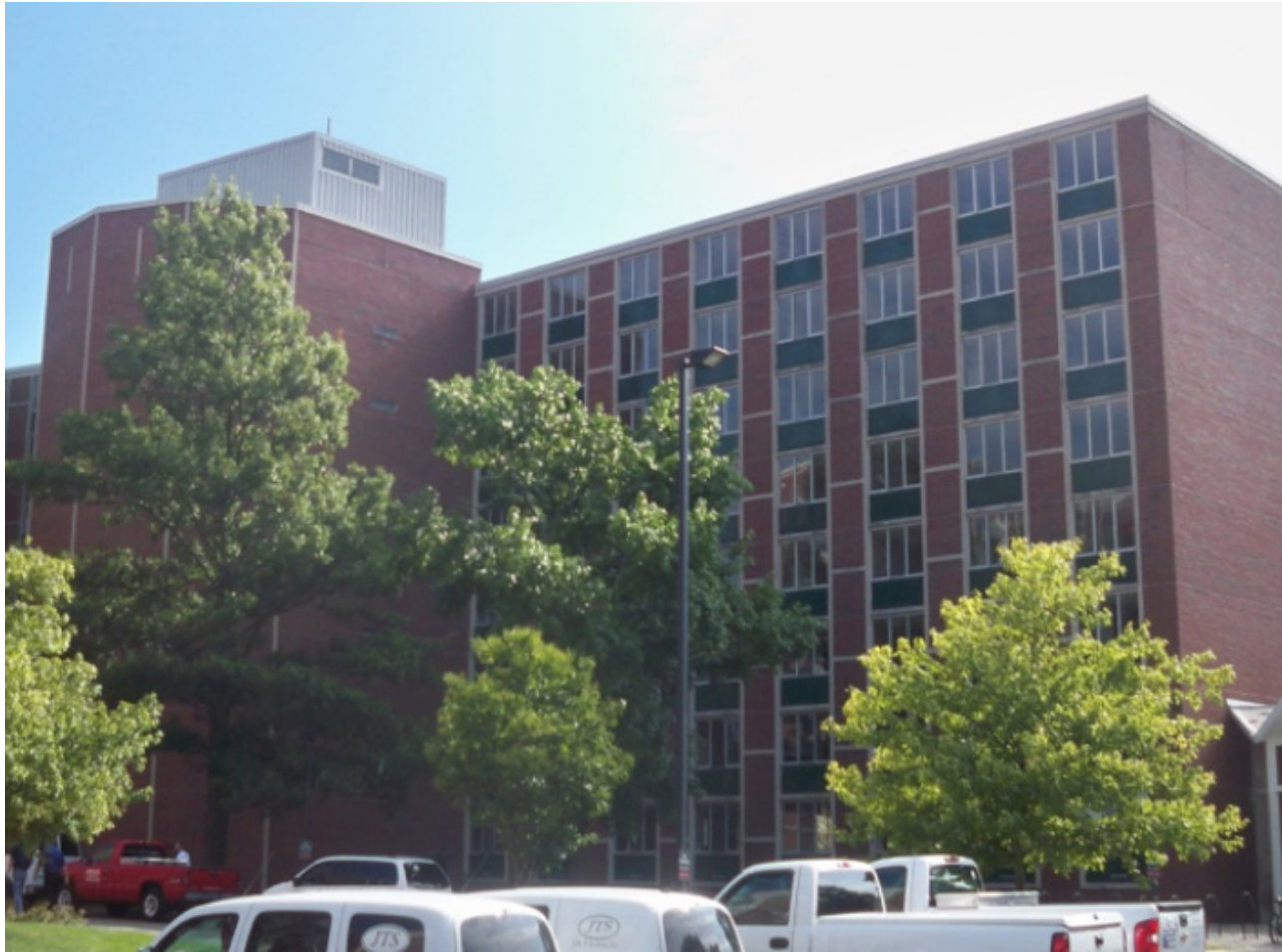
BALL STATE UNIVERSITY - STUDEBAKER DEMOLITION
