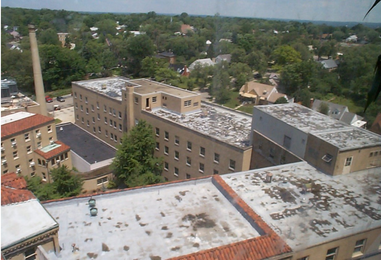
GOOD SAMARITAN HOSPITAL- MADONNA AND EAST WING DEMOLITION
