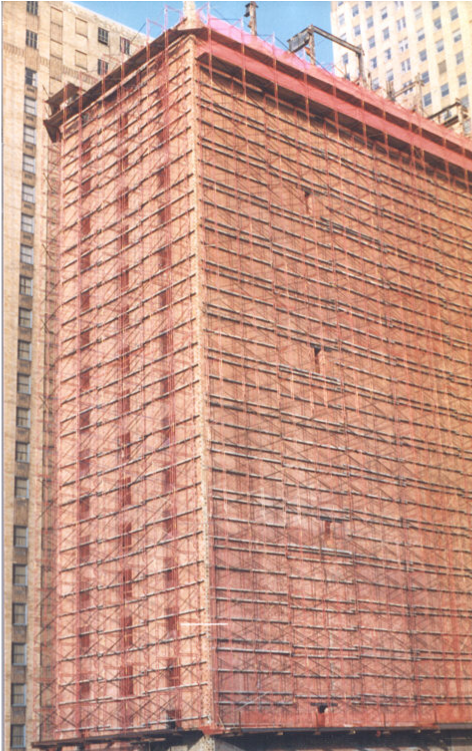
CAREW TOWER PARKING GARAGE DEMOLITION
